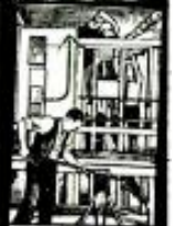
HOUSE WIRING only one of the many branches you "Learn By Doing"
